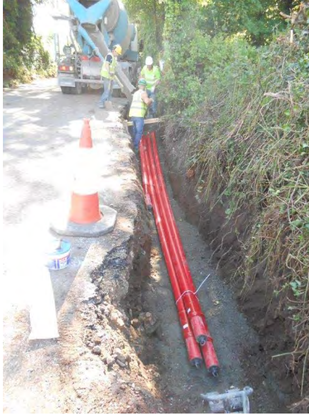
Plate 2.2: Cable Laying, Trefoil configuration
