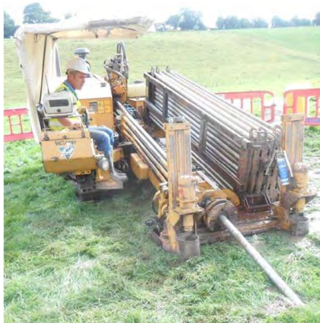
Plate 2.2: Horizontal Directional Drilling under the River Blackwater in County Cork, August 2014
